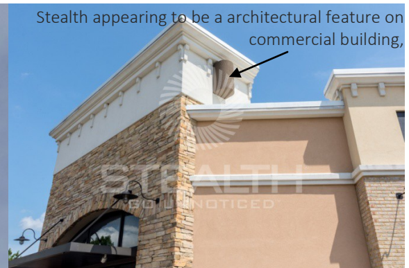
Stealth using a Cupola Feature
