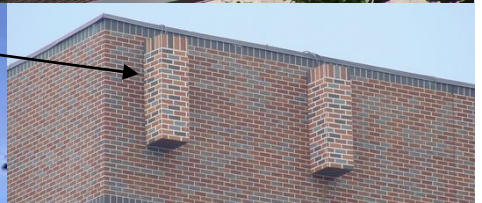
Stealth using a Chimney Concealment in Goleta, CA
